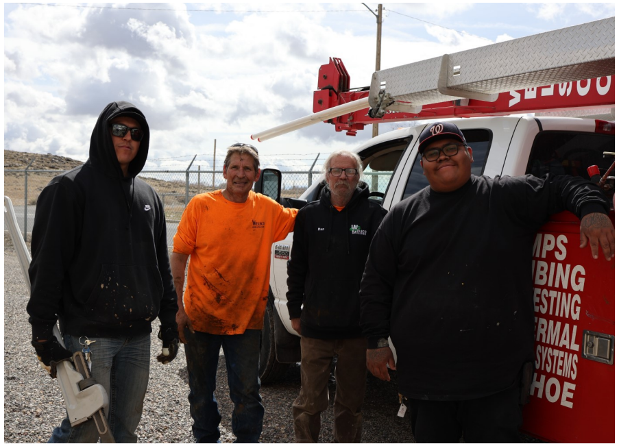
Public Works & Welsco well pump replacement
